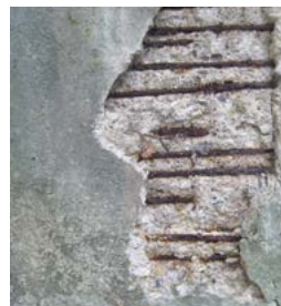
Ill. 2: Steel corrosion
